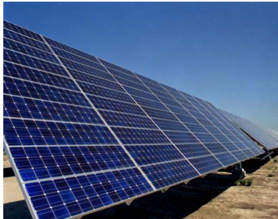
Diodes and PV cells are both devices made from P-type and N-type silicon that allow electrical current to flow in one direction only.
